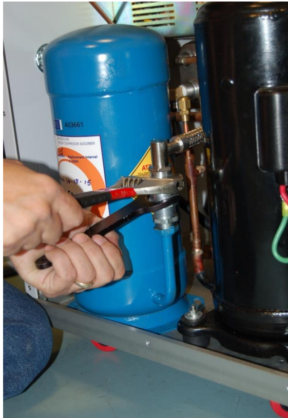
Figure 7 – Adsorber Aeroquip OMS Supply Line Removal
