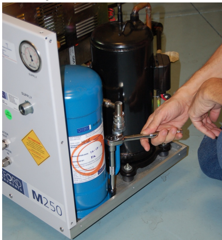
Figure 9 – Adsorber Chassis Screw Removal
