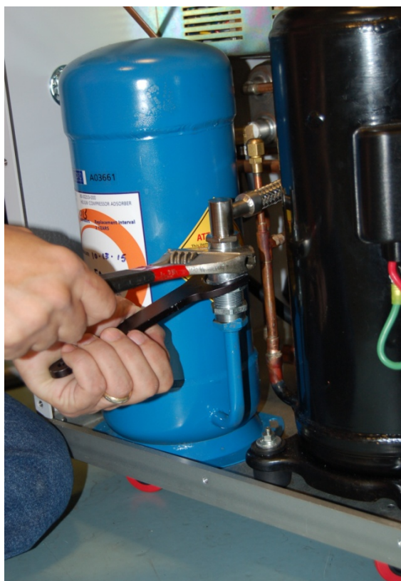
Figure 7 – Adsorber Aeroquip OMS Supply Line Removal
