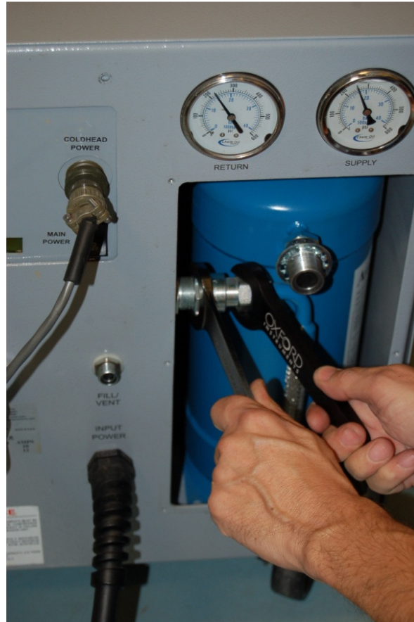
Figure 16 - Adsorber Aeroquip OMS Supply Line Removal
