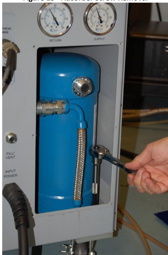
Figure 15 - Adsorber Screw Removal
